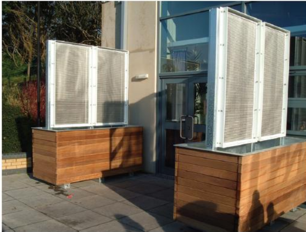
Figure 4: Screens, incorporating planters, used to provide local wind protection at a windy entrance
